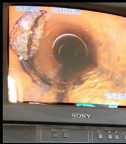
A resident on Court Avenue has been having wastewater issues. Upon inspection, the lateral connection protrudes into the side of the 6" terra cotta main line by over an inch. The camera was not able to pass by the protrusion. The mainline was also cracked and in danger of falling apart. It was decided to install a new section of mainline and replace the lateral.
