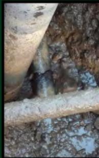
The cast iron connection most likely was causing the blockage along with a possible reverse flow issue. There was also a severe crack in the transite portion of the lateral.
