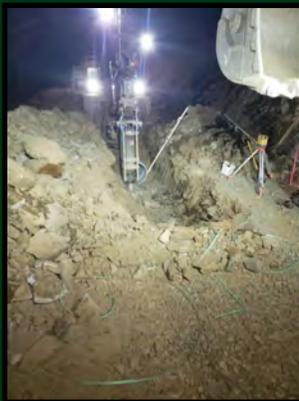
With current fire restrictions in place, the USFS was able to grant a waiver so that the PW Mountain Line crew could continue work installing the 24" pipeline in the ground. This will allow the reconnection to the existing line happen as soon as possible. The crew has been allowed to work the hours of 4:00am to 1 pm with a one-hour "fire watch". Two fire suppression trucks are onsite at all times and available for use.
