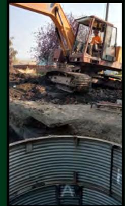
The wastewater excavation work on Birch Street was backfilled and completed on Tuesday of this week. Last Friday, 38' of 8" PVC pipe was installed at a depth of around 12' to supply service for the new homes planned at the Silver Birch subdivision development. Excavation conditions were very difficult with groundwater filling the bottom of the deep trench and the sides of the trench sloughing off into the excavation.
