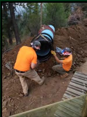
Left: Scott and Riley work to attach one of the last ductile iron angle point fittings to the pipe near the tie-in point. Once the old concrete line is connected to the newly installed 24" PVC line, water from Salmon Creek, Little Salmon Creek and a few small natural springs can once again be brought to Baker City for municipal use.
