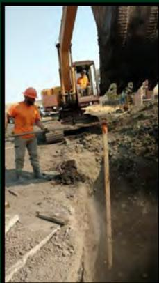
The line was installed successfully and a long 2" x 4" placed at the end of the pipe so that the contractor will be able to follow the board down to the end of the pipe when they begin their portion of the work.
