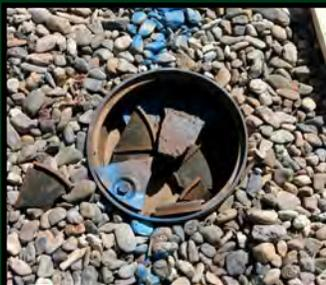
A local contractor contacted Public Works on Thursday to request a new lid be installed where a concrete delivery truck had driven over and broken a water meter lid.
