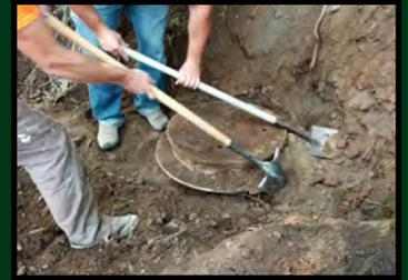
Baker City Public Works assisted the City of North Powder last Friday and Saturday to locate a manhole which had been buried for many years, so that the line could be cleaned and to remove wastewater blockages.
