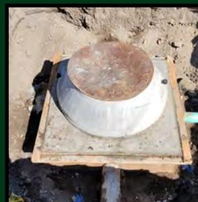
After the concrete had cured, the tops of the PVC pipes were cut out to allow for cleaning and inspection work.
