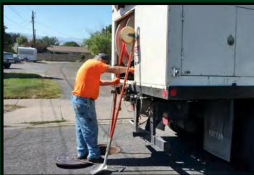
One particular wastewater line in town has been requiring quite a bit of time to keep it flowing properly. This 6" diameter concrete line is only 130' long and only has three houses connected to it. Yet, it needs to be cleaned once every six days to keep it from plugging.
