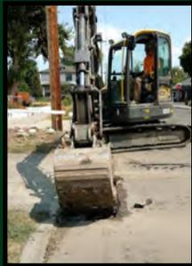
Hot asphalt was used to repair the street gutter line on "A" Street between Main and 1st Streets. The existing asphalt along the curb had deteriorated to the point where it needed replacing.
