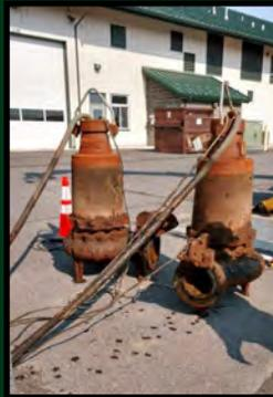
Public Works was able to assist ODOT in the removal of two pumps from their wash rack wastewater vault.
