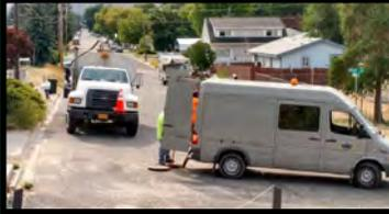
Karl and Rick responded to a call about a plugged wastewater line. The video-inspection camera was used to navigate the problem and the jetter was brought to the site in case there was a plugged main line.
