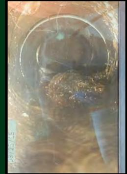
A root ball was the cause and a professional drain cleaner was able to cut it out of the line.
