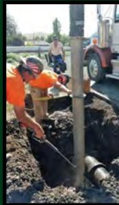
Next a bell clamp was attached to the connection to keep the leak from reoccurring. The concrete curb will be replaced as time allows.
