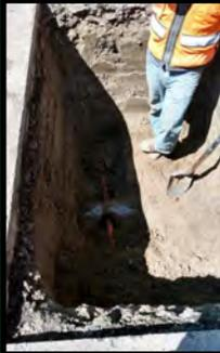
A recently installed fiber optics line damaged a city stormwater line.
