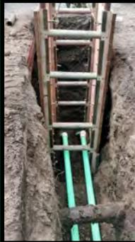
Left: The parallel wastewater laterals were successfully installed.
