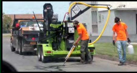
The new combination crackfill and mastic patching machine is working very well. Crews worked to fill cracks on several blocks of streets which will be chipsealed starting August 17h.
