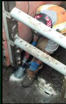
Left: Nate core drilling the new lateral attachment.
