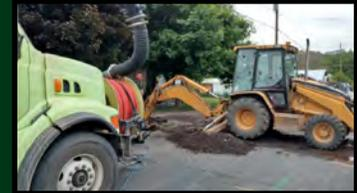
Right top: The backhoe and Vactor truck were used to excavate the trench.
