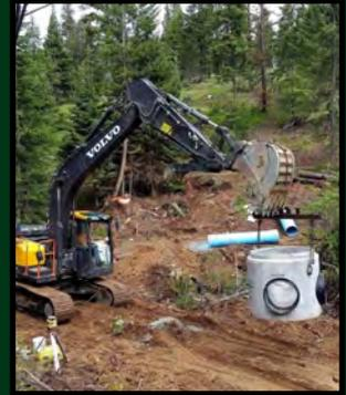
The first precast manhole was successfully set into place on Monday. The manhole has three rubber boots, two 24" and one 8" for pipe connections.
