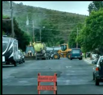
Left: The asphalt surface was demolished using the “zipper” and Volvo loader.
