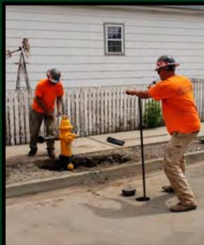
The valve in the street was turned to the off position, the location was hydro-excavated and rusted connecting bolts were removed along with the support blocking.
