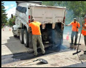
Public Works patched several trenches this week using hot asphalt. Here they are working to patch water line trenches on Court Avenue.
