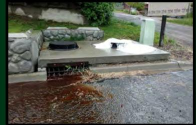
Right: Stormwater was flowing into the sediment vault on Auburn Avenue as designed. The vault was installed several years ago to intercept sediment and debris before it can flow out onto the city street. The vault was cleaned Thursday to remove sediment.
