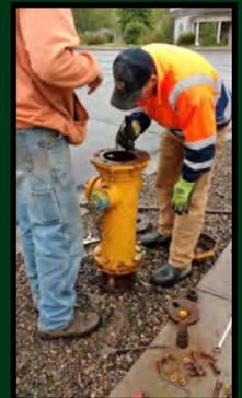
Far right: Justin and Brian worked to repair the fire hydrant on Orchard Street. It was determined that the hydrant could not be economically repaired. It is currently out of service and is scheduled to be replaced.
