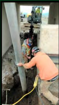
Left: At the Water Reservoir, Scott, Blain and Nate worked to install a new water sample line that runs from the Goodrich pipeline to a pump that is located inside an existing vault. Heavy rains made the work difficult. Because of safety concerns, the project was rescheduled to next week.
