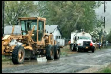
Left: Stormwater work was performed on 2nd Street in South Baker. Two shallow storm lines were cleaned and sections of a drainage ditch constructed.
