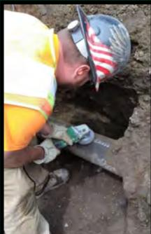
Left: Photos from the 6" water line. Embossed lettering on the old cast iron pipes had to be ground off so that the stainless steel tapping sleeve could form a water tight seal.
