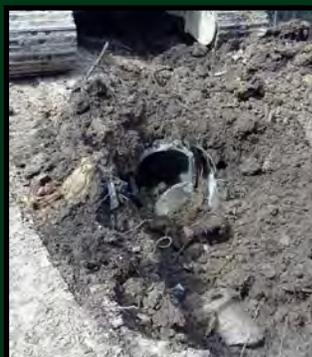
The old undersized concrete pipe is visible in these two photos.
