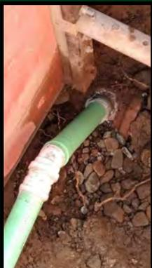
A special ABS to PVC adapter, coupler and cement was used to secure the connection.
