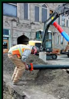
Left: Here Nate is installing the rubber gasket and 6" mega-lug fitting.
