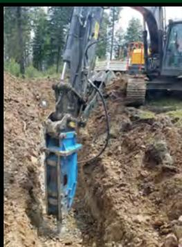
Progress is going well on the installment of the new 24" water line at the Elk Creek Settling Tank to Salmon Creek Mountain Line project. Difficult digging was encountered through one of the recent sections.
