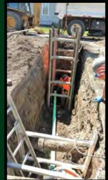
The line that was replaced consisted of Orangeburg pipe and was beginning to fail.
