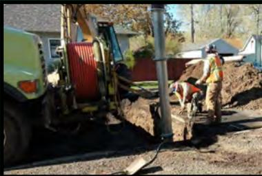
The asphalt surface was "zipped" using the Volvo loader with zipper attachment.
