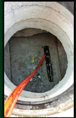
Karl entered the manhole to cut the top of the Orangeburg pipe while Tom was the attendant. The atmosphere was constantly monitored for safety. As you can see, the oxygen content was 20.9%. The wastewater vault which is now located on the west side of Clark Street was used to access and clean the line. A blockage at 36' was temporarily removed using the jetter and a high pressure water stream. The line was then video-inspected and determined to be in poor condition.
