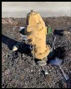
The Fire Department personnel noticed that the fire hydrant at the intersection of 10th and H Streets was leaning awkwardly. Upon inspection, it was discovered that it was struck, most likely by a vehicle, and the water supply pipe was broken underground.
