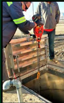
The contractor, the lift manufacturer's representative and Baker City's contract engineer gathered at the new "H" Street lift station to go over operation & maintenance procedures with Public Works personnel. The new pumps in the wet well vault are 3-hp submersible pumps attached to a sliding rail system.
