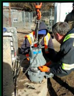
Right: Here you see where the pump slides between the two rails for easy removing during maintenance procedures.
