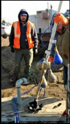
Left: These are the floats which sit near the bottom of the wet well. As the fluid level in the vault rises, the floats change orientation and cause the pump(s) to automatically turn on. Then as the levels drop, the floats again change orientation causing the pump(s) to turn off.
