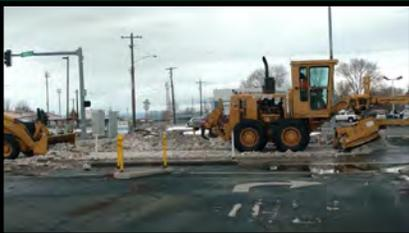
Temperatures warmed up enough that the remaining snow berms could be broken up using the CAT grader and backhoe. Justin and Blain shaved off portions of the berms into smaller pieces so traffic could further break down the snow. By days end, the berms were completely gone.
