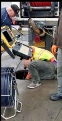
Left: The push-cam was used to inspect and locate the end of the line.
