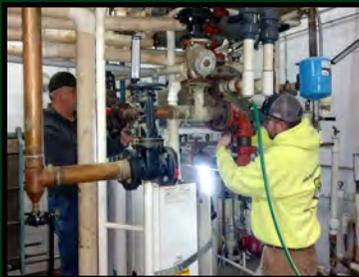
Preliminary work was done this week on the repair to the heat exchanger unit in the mechanical room. Dismantling the old and corroded pipe proved to be quite a challenge.
