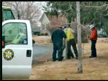
Tommy and Riley assisted OTEC with the hydro-excavation of buried power lines which supply power to the street lights on Kirk way.
