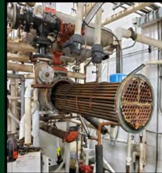
Right: Here the heat exchange unit for the pool has been partially removed from its vessel.
