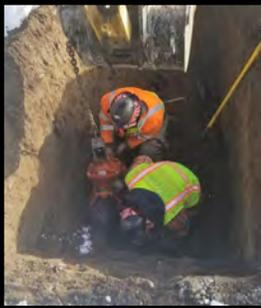
Public Works has been involved with the new Park Springs development near the Sam-O Pool. A new 6" water valve was installed near the south edge of Baker Street so that the developer could install a 6" x 8" adapter near the valve, then lay 8" ductile iron pipe to serve the subdivision lots.
