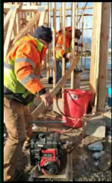
Public Works in conjunction with the Baker City Fire Chief worked to pressure test the 6" fire line that was recently installed at the New Directions Northwest complex. Blain and Brian pressurized the line to 200psi of water pressure. The pressure held and the test was approved by Chief Clark.
