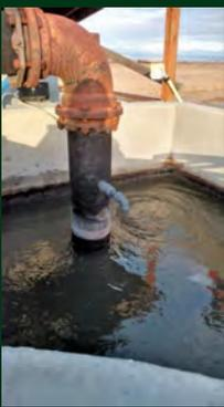
There have been some problems with the lift pumps becoming partially plugged recently. When wet wipes and other items become entangled within the pump mechanisms, it causes them to be inefficient. Rick, Karl and Jake worked on the pumps several times, with some success, to clear the blockages.
