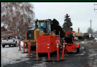
The contractor has begun excavation work at the "H" Street lift station site. Bypass float system, generator and pump are in place near the intersection of 8th Drive and H Street.
