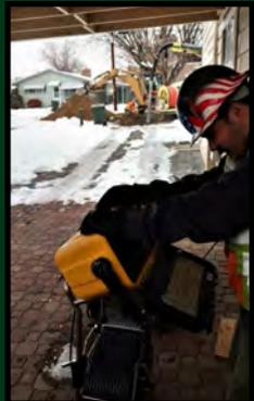
Left: Jake and Riley assisted with the project by video-inspecting the remaining lateral from the house to the street.
