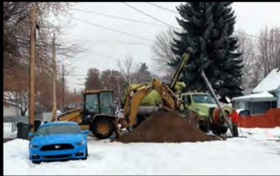
The asphalt was pulverized using the Volvo loader and rented asphalt zipper unit.
