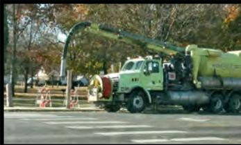
Two new bollards will be installed at the northeast corner of the Geiser Pollman park to deter unauthorized vehicles from driving through the park. The vactor truck was used to hydro-excavate for the bollard placement.
