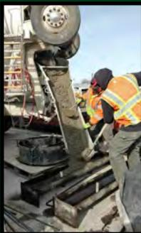
Three cubic yards of concrete were poured on Thursday. The pour included two park bollard bases, three eco-blocks, two wheel stops, nine thrust blocks, one 12" lift ring and one 2" lift ring.
