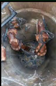
Problems continue to occur at the "H" Street left station. The pumps lose their prime regularly. When that happens, the pumps are unable to begin pumping wastewater out of the wet well. Water from jugs is used to prime the pump.
