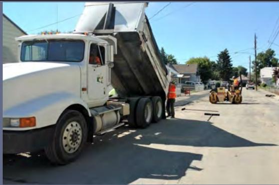
Asphalt patching was completed on Clifford Street on Friday. This work was the final step in the completion of the new water main line project.
