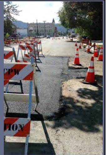
The Washington Street Main Line Bore Project was completed this week. The crew patched bore holes on both the east and west side of the Powder River along with a water trench line.
