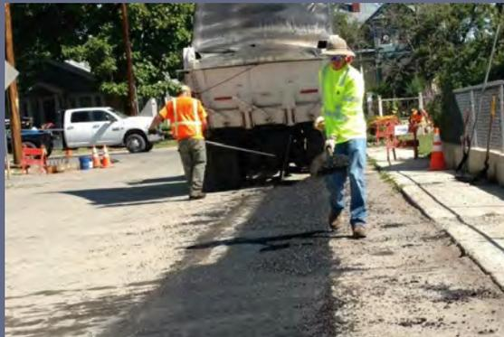
This patch was intentionally left low because the existing asphalt in this area is too high and will be ground down next week.
