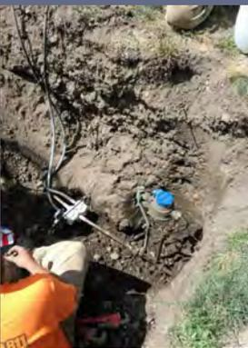
Blain and Nate were able to freeze the charged service line to stop the flow of water so that a new meter setter could be installed.
