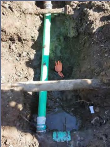
Left: Last Friday, while a contractor for Cascade Gas was working on Madison Street, they noticed that a sewer lateral was leaking. Blain, Karl and Nate verified the leak and worked after hours to replace the pipe and repair the leak.
