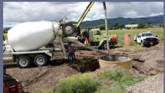
Right: Concrete was poured around the connected piping within the manhole shielding.
