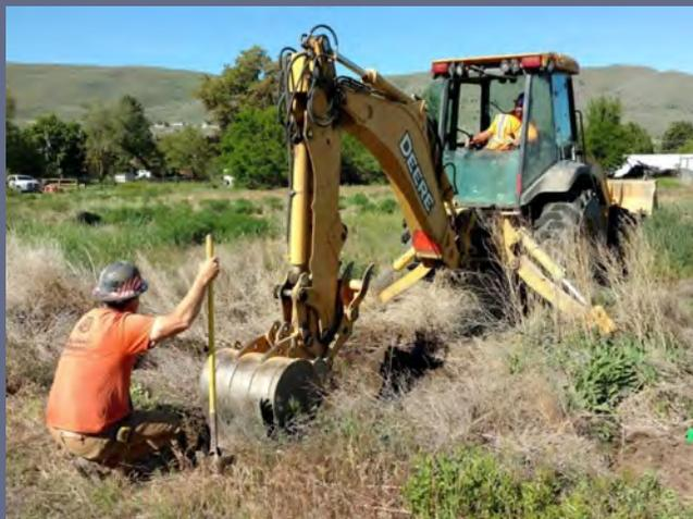
Blaine and Tommy installed a new water service on 11th Street this week. The line replaces a 1” copper service line that was installed in 1979, just prior to 11th Street being constructed.
