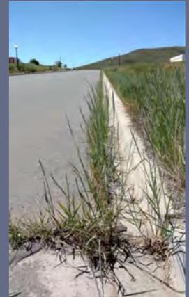
To the left, you can see settlement that will need to be filled in. Crews will use a "D" mix asphalt to make the repairs.
