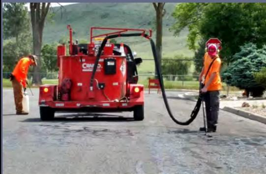
Public Works Crew began filling in cracks on streets this week in preparation for the 2019 Chipseal project. Heavy grass growth will be removed so that the curb line can be filled in prior to the chipseal application.
