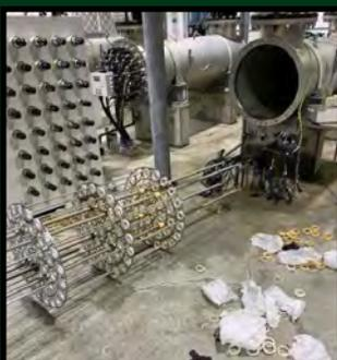
Left: A broken sleeve was discovered in the #3 UV Vessel at the reservoir on Friday. It was removed and replaced, along with wiper blades.
