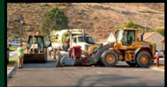
The 4-person crew made excellent progress this week installing the new 24" PVC water line along the "Pipeline Road". Nearly 500ft of line was installed Thursday including three ductile iron angle fittings.
