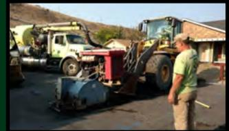
Right two: New water and wastewater services were installed in the 1600 block of Balm Street on Thursday. Asphalt was cut and both services were completed by the end of the day.
