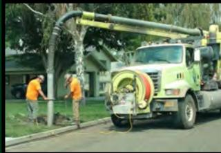
Left: A water leak on 9th Drive was repaired using the Vector truck.
