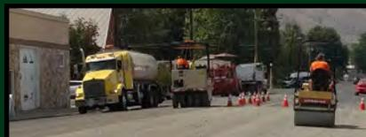
Bottom three: Reservoir Road was chip sealed Wednesday morning. It is a steep road and special attention must be taken so that tires do not "spin out" on the slick oil and rock mixture.
