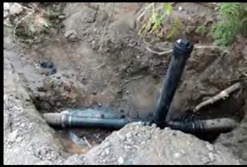
A professional drain cleaner reported an issue with a wastewater lateral in an alley south of Auburn Avenue. The owner had excavated down to the lateral and a plumber had installed a cleanout. The line was still unable to be opened. Public Works will inspect the main line early Friday morning and determine the cause of blockage.
