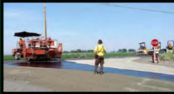
The last street of the day was 9th Street from Hughes Lane going towards "L" Street. The remaining oil in the distributor's truck was used on this stretch of road to preserve the asphalt grinding base.
