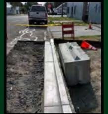
A new low curb was constructed on "C" Street between 10th and 11th Streets. A Huge 3,500 pound concrete block was placed behind the curb to prevent it from moving while the hot asphalt was being placed next to it. Normally asphalt is patched after the ramp is complete, but in this case it was patched first for efficiency.
