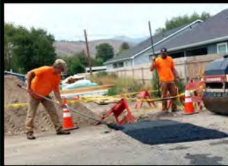
Here the crew is working to patch 10th Street on the truck route where two wastewater laterals were installed for a new duplex.
