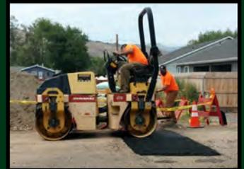
On Reservoir Road, a structural fabric called glass grid was used to help keep the thin chipseal surface from continuing to crack and form potholes. Once the area is premeasured, the fabric was peeled from a roll and cut to size. It was then placed over fresh tack oil and pressed onto the surface. It was then covered with fresh, hot asphalt and compacted with a steel wheel roller.
