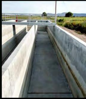
The discharge of treated effluent from the Wastewater Treatment Facility ceased this week. The chlorine contact chamber was thoroughly cleaned and prepared for when conditions improve and discharge begins again.
