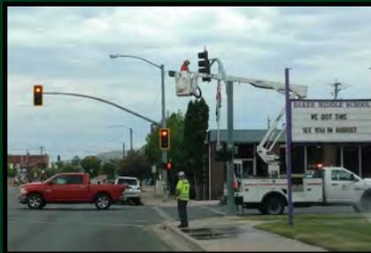
ODOT installed bright reflective borders around some of the traffic signal lights.
