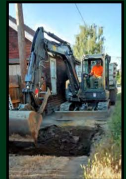
A resident on Second Street reported that their wastewater line was plugged. An emergency underground locate was called in immediately. Public Works used the push cam to locate where the lateral goes from a cleanout near the house with the plugged line.
