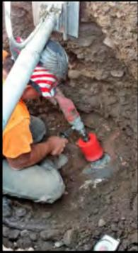
A wastewater lateral was relocated for a house on 2nd Street earlier this week. Here, Karl is taking the steps for the installation of the new lateral by installing an Inserta-T connection.
