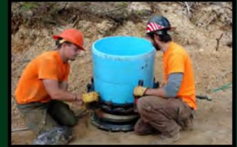
Specific fittings are bolted together to provide the necessary deflection for proper alignment. Trace wire and electrical conduit are installed for future use. A rotating laser level helps the crew maintain proper grade. A big THANK YOU to the Baker County Road Department for the use of their CAT dozer to help with the installation of the project.
