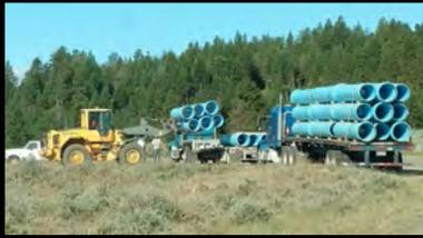
Several truckloads of 24" heavy duty PVC pipe were delivered and unloaded. It is scheduled to have this entire stockpile installed and in operation before winter weather begins.
