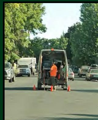
A wastewater lateral problem occurred on 4th Street, where laterals from two homes were connected together (this is no longer allowed). Karl and Jake video-inspected the lateral and main line connection. The property owner hired a local contractor to install a clean-out between the curb and the sidewalk so the plugged line could be cleaned.
