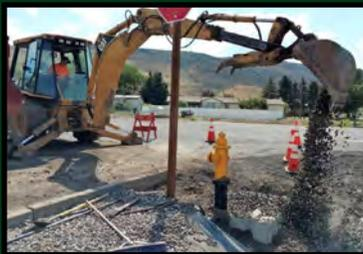
Justin and Brian installed a new fire hydrant to replace a broken hydrant near the intersection of Hwy 7 and Colorado Avenue.
