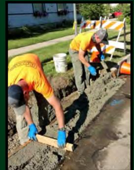
Blain excavated the old section of curb so Kris and Matt could construct the new ADA compliant curb.
