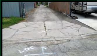
"C" Street between 10th and 11th is scheduled to receive a Chipseal treatment this August. This concrete alley approach will need to be repaired before that happens.
