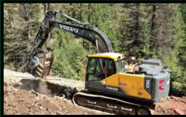
Brian uses the crusher bucket to create bedding for the new 24" heavy duty PVC pipe.
