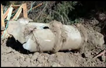
Crews continue to make excellent progress on the new 24" mountain pipeline project. The old non-steel reinforced concrete pipe was susceptible to tree and grass roots entering into the broken pipe and slowing water flow to town. Justin discovered that one section of the old pipe had the bottom broken and probably had been leaking for many years.
