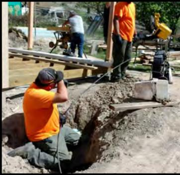
Karl and Jake performed a video-inspection of a private wastewater lateral on Auburn Avenue. The line was located and determined to be in excellent condition. The plumber was billed for the work.
