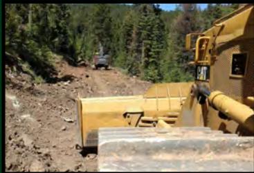
Left: Once the pipe is installed, bedded, backfilled and compacted, the CAT dozer smooths out the road surface.
