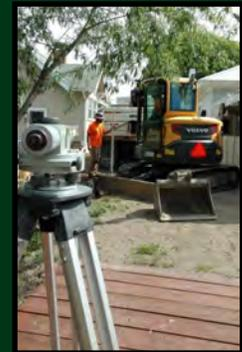
Blain and Nate replace a portion of a stormwater line that runs between two properties on Orchard Street. The line was plugged with massive roots and mud. The pipe elevation was measured to verify it would drain properly.
