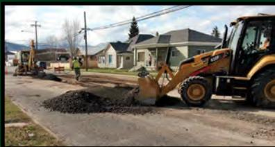
Left: A new 1" water service was installed on Oak Street for a new building near the Campbell Street intersection. Justin, Brian and Nate performed the excavation and installation work.
