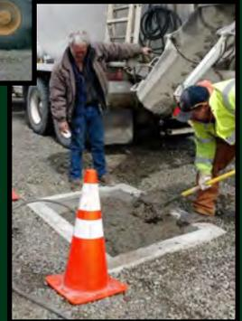
Here you see the prepping of the manhole vault and setting the vault over the 30" pipe. Scott and Tom placed concrete around the pipe to form a monolithic mass. The top of the pipe will be cut out next week to provide access for maintenance.
