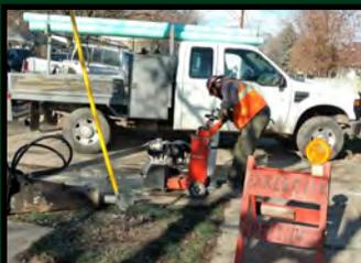
Work began to replace a wastewater lateral which extends across Auburn Avenue just west of 4th Street. A concrete flush vault had to be demolished and a concrete alley approach had to be sawed out with a portion of it being removed. Blain began excavation.
