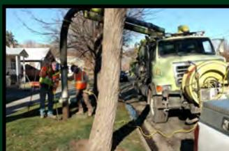
Brian and Riley hydro-excavated down to the elevation of the existing lateral near a clean out. The elevation of the pipe was then measured to determine the necessary slope of the new 6" PVC pipe.
