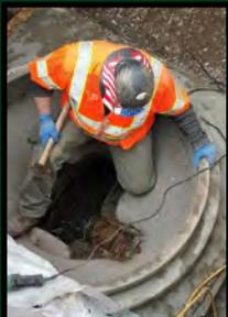
Left: Karl cutting the tops of the two pipes to provide access.
