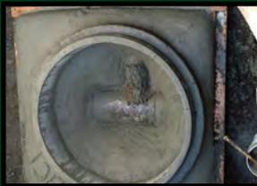
The manhole on D Street between 5th and 6th Streets was completed earlier this week. The tops of the terra cotta and orangeburg pipes were cut out and the 6" orangeburg pipe going North was video inspected for 90'.
