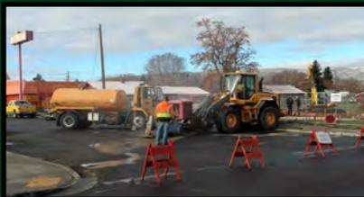
Left: The final main line connection on Court Street has been made. Several remaining water meter connections will have to be made this month. Because of recent precipitation, the street has become rather muddy. Clean-up work will continue until the street surface is acceptable.
