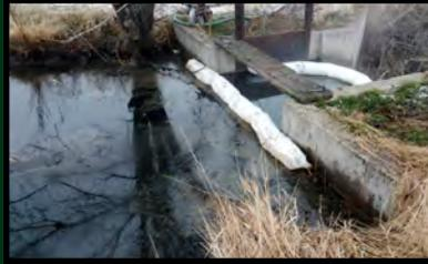
Petroleum clean up work continued this week on the New Home ditch. The surface film was removed using the vector truck and new absorbent booms were installed.
