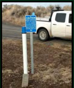
This cathodic protection and blow-off station up Alpine Lane was raised to grade as shown. The “C” and “B” identify the structure as “cathodic protection” and “blow-off”.
