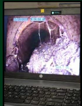
Above right: Video inspection revealed heavy root intrusions entering thru the joints in the 8" concrete pipe.
