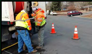
Karl and Rick operated the jetter with the root saw attached to cut the roots from inside the pipe.
