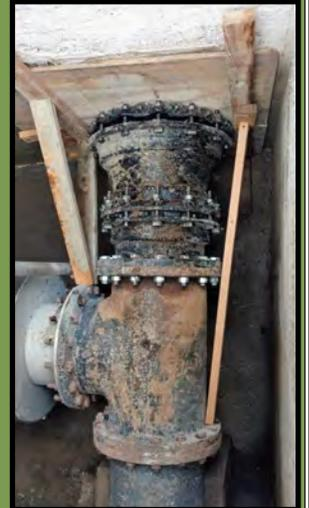
A larger hole had to be cut into the Elk Creek settling tank wall for installation of the new 20" ductile iron pipe.
