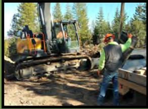
The 20" valve weighing approximately 1,500 pounds was successfully installed Thursday along with the remaining pipe necessary to connect to the 20" ductile iron line.
