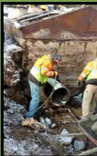
Once the hole was cut and the pipe penetration complete, pre-mix bags of concrete were used to seal the connection.
