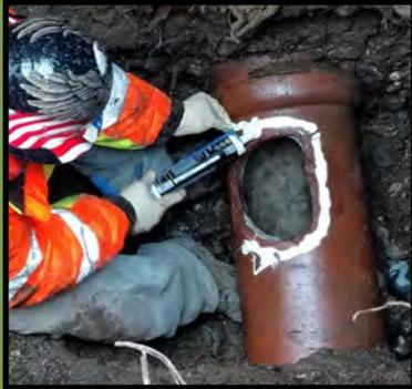
Roots were the cause of a blockage. A special insert-a-tee connection was used to attach into the 10" CIPP lined pipe.
