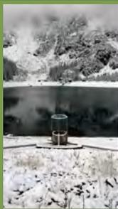
Winter-like weather was the theme at the beginning of the week at Goodrich Reservoir. The crew of Justin, Blain and Brian worked on the Goodrich Reservoir repair work most of the week. 40" of 48" squash pipe was hauled to the site and installed to protect the outlet discharge point.
