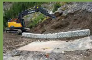
Blocks were stacked with a layer of fabric between each horizontal layer. Existing seepage drain lines were plumbed together with the outlet of the hose ending near the west end of the new retaining wall.
