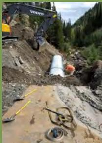
The pipe was carefully placed against the sharp crested weir located under the steel plates. The next 2 20' lengths were banded together and covered with appropriate fill material.
