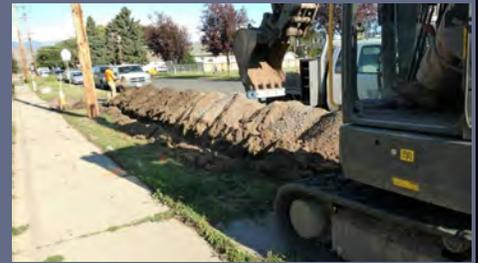
Right: A resident was without water this week because their line running from the meter to the house had developed a leak. As soon as Public Works became aware of the problem, an emergency locate was called in and the meter was re-located to its proper position in front of the house being served.
