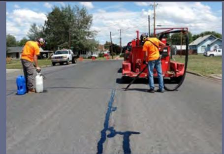
Several members from Public works have been involved in crack filling the streets this summer. Jake and Riley, along with summer workers Cayn, Dylan, Caden, Hunter and Zach have all taken turns filling in cracks on Baker City streets. Here they are working to fill cracks on "D" Street between College and 10th Street.
