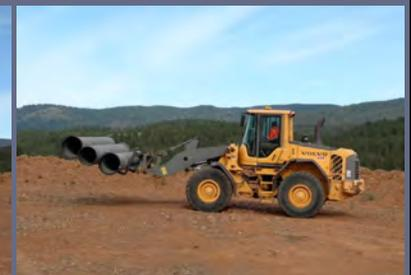
Justin and Scott unloaded the first trucks. Each piece of pipe weighs approximately 1,890 pounds. Justin used the Volvo loader to perform the work.
