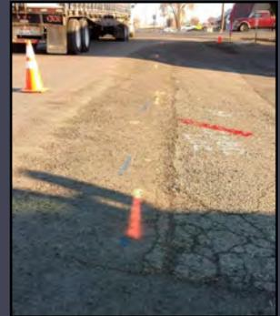
A representative from the fiber optics utility company, MCI, had to travel from Boise to mark the location of their line. As you can see in the photo the fiber optics line runs directly in line with the 10" water main line. Fortunately the fiber line is located under the water line so it was not disturbed during the water line repair work.
