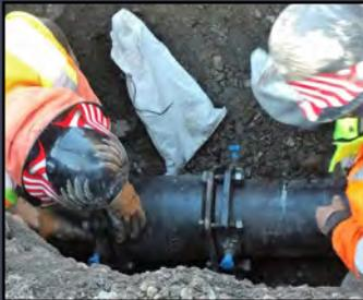
Here you can see that the "solid sleeve" fitting is properly attached and locked into place with no leaks. The blue "locking" bolts are tightened to the point where their top simply snaps off the shaft part of the bolt. This verifies that the bolt was tightened to the proper torque to lock the sleeve into place.
