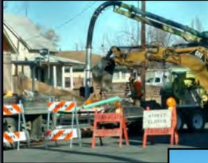
Karl and Riley working to remove a portion of the old concrete lateral and install a permanent plug so roots and ground water will be kept out.
