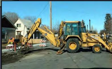
Riley operating the Backhoe with attached compactor to complete the backfill process.
